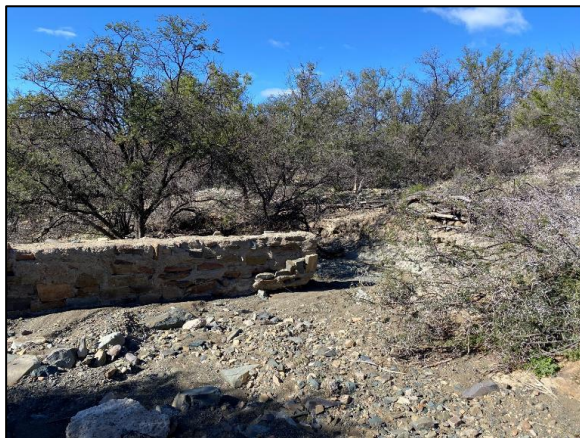
Figure 22: Several small weirs were found within the steeper valleys through-out the study area, most no longer functional
